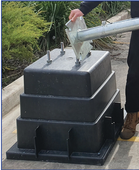
Fig. 2.3a Mounting pole onto concrete base
