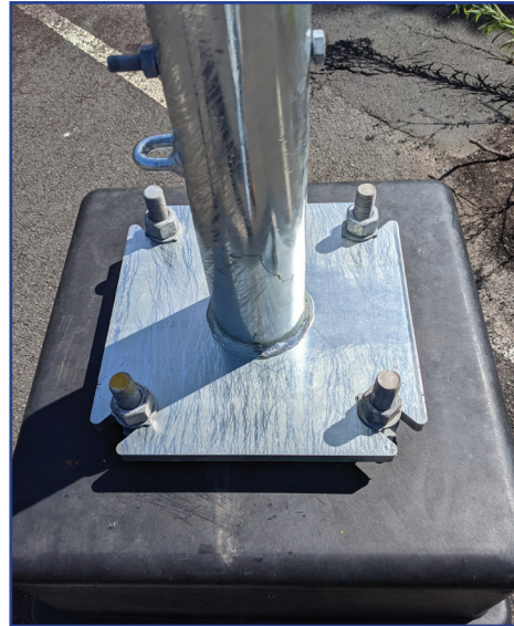
Fig. 2.3b Pole fixed onto on concrete base
