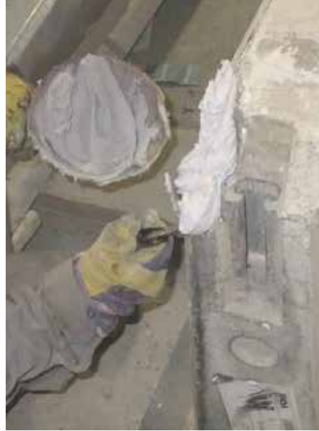
Application of Sikadur-31 adhesive
