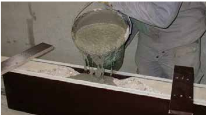
A makeshift formwork is prepared before pouring SCC concrete or grout
