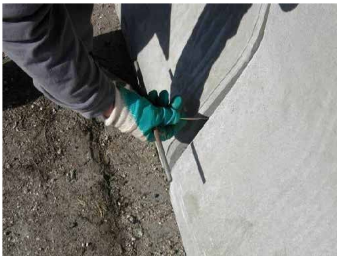
Mounting of a butt joint insert
