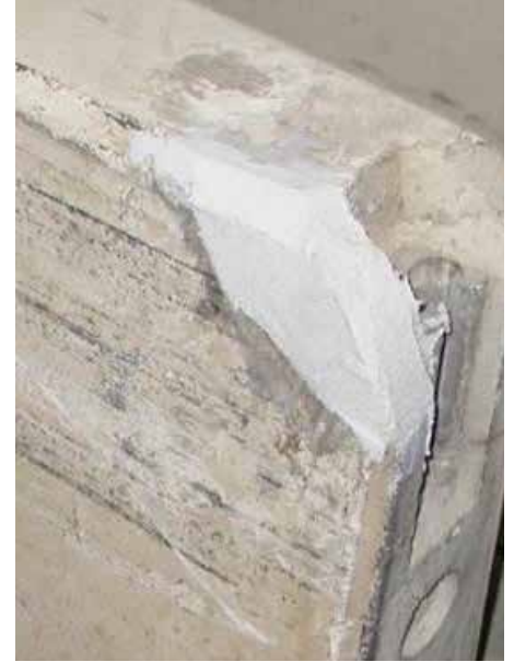
Result of step 1: rough shape
