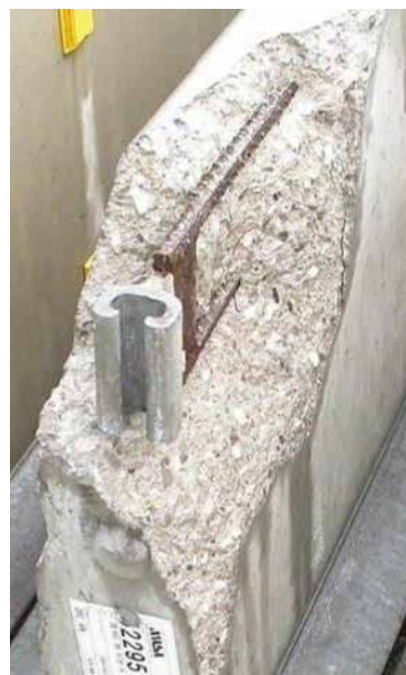
Tension bar has been completely exposed
