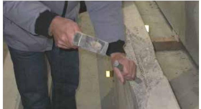
Chipping off loose concrete and cleaning of breakage surface
