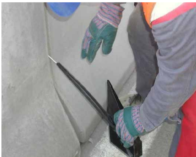
There is a worker on each side pulling the elastomer strap using a metal hook
